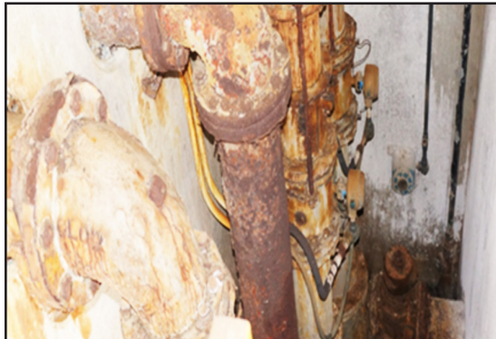
Corroded pipes
